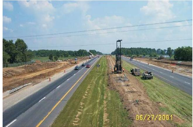
Figure 2. Holes being drilled for grout injection into abandoned mine along I-77 in Summit County, Ohio.
