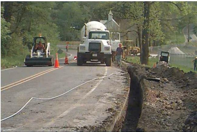
Figure 3. Installing coaxial cable in the trench along SR91 in Plasterco, Virginia.
