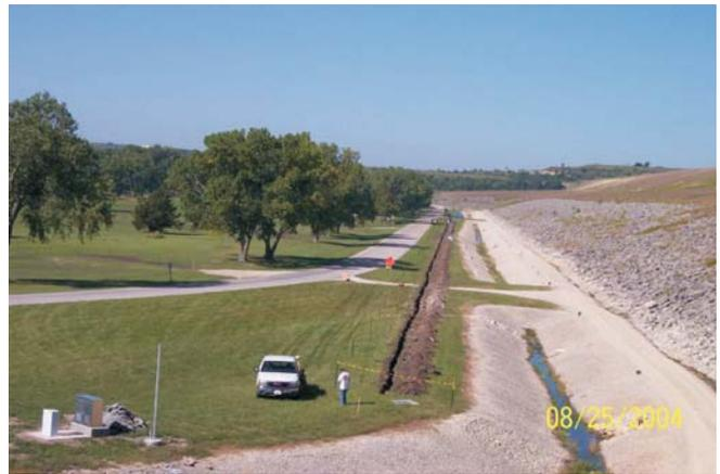
Figure 4. Installing coaxial cable in the downstream trench at Tuttle Creek Dam in Manhattan, Kansas.
